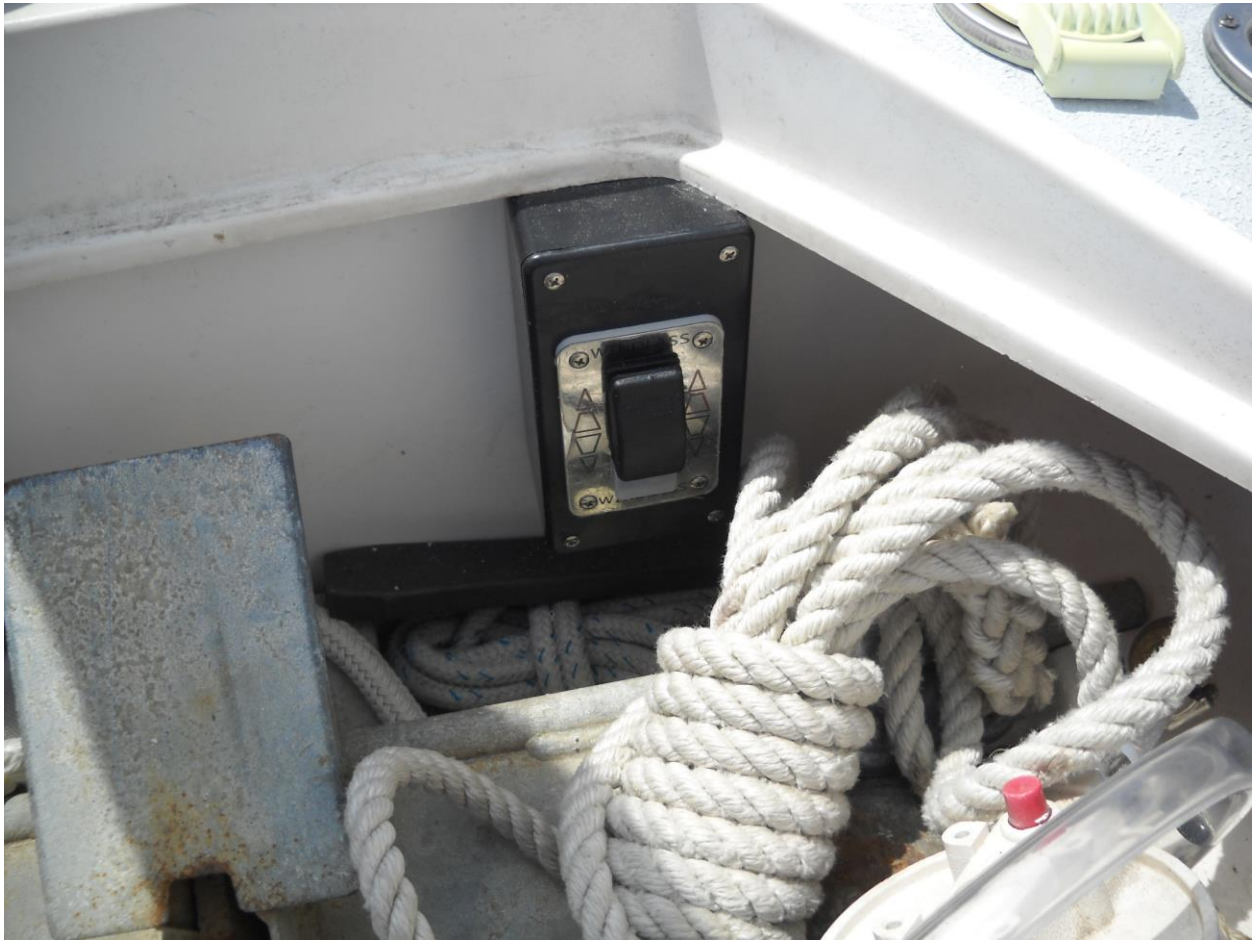
Up/down switch in anchor locker
