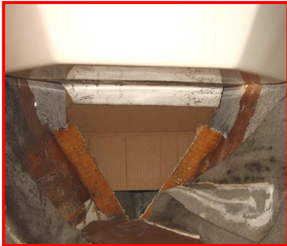
I duct-taped heavy cardboard to provide the FB wall backing, knowing that I could rip it off from the inside once the whole thing had cured.
