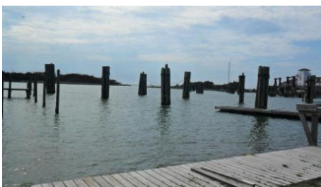
Pier at the state park
