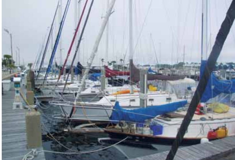
The Panama City Marina docks overlook wide-open St. Andrew's Bay and its Gulf inlet but offer full protection via a massive concrete pier and breakwall.
