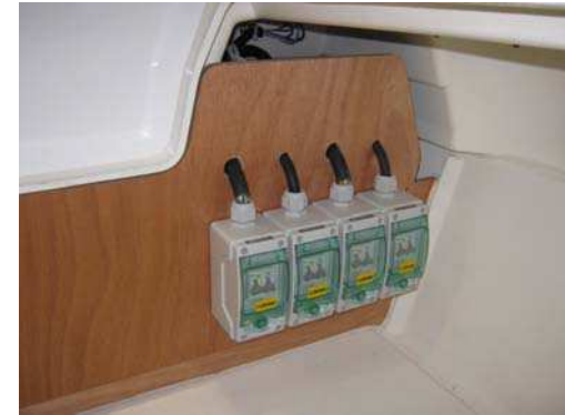
Bipolar circuit breaker 32A (Ref 2)
