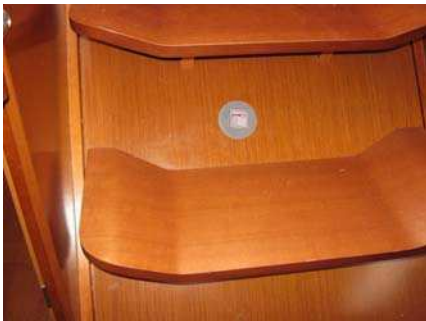
Extinguisher hole located under the companionway step
