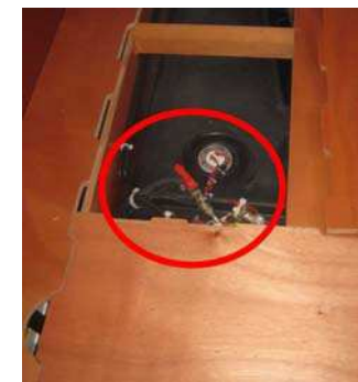
Supply valve Extra tank (Ref 1)
