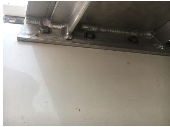
Bolted connections complete
