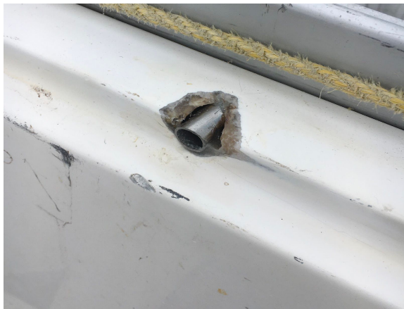
Repair with epoxy fill and stainless tube insert
