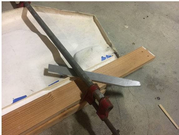
formwork for ledge on operable lid section
