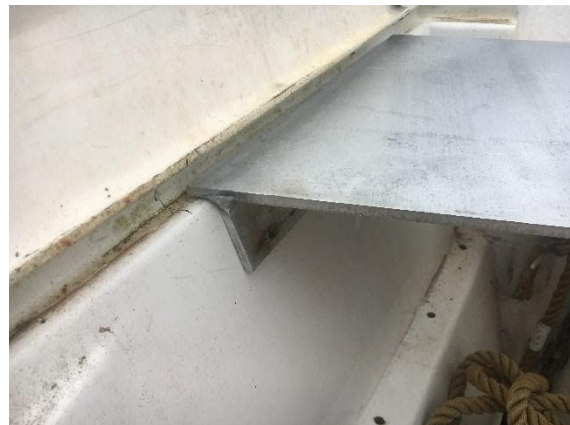
Test fit after welding
