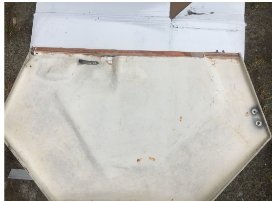
Epoxy fill at support ledge
