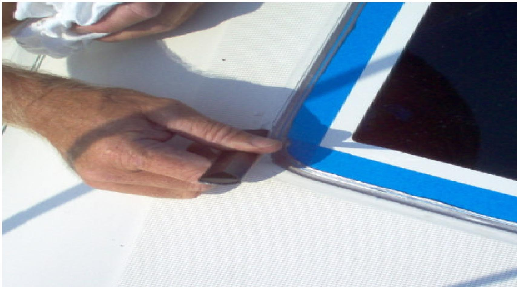
Remove excess sealant
