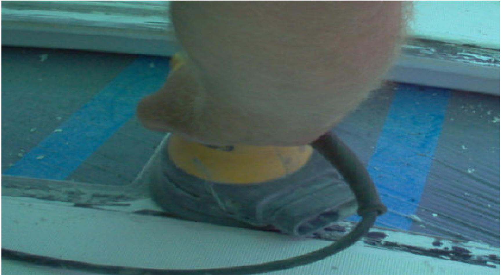
Remove the old adhesive. Vacuum and prepare for pre-fit
