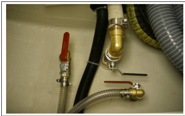
Figure 23: Rapid shut off valve shower room
