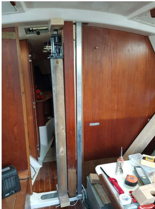
The header was placed with gobs of epoxy on top, and held in place with one of my bottle jacks to set. It was not easy getting it square and level, and in the end I had to do a bit of shimming between the header and the post to support it evenly. The newspaper is to keep any epoxy from dripping on the teak bulkhead.
