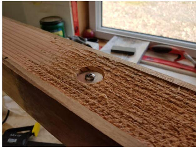
Now I could glue the front face back on, and need only a wood plug for access to the screws, leaving the washers buried inside. If the post ever needed to come out it could be removed by just taking out those three screws. Any future owner had better have a copy of my maintenance log, or they're going to have a pretty tough time trying to figure out how to get that post out if they ever had to...
