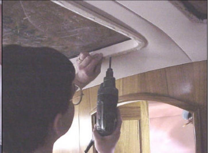
Secure ring in place using #8 x 3/4" beige truss head screws.
