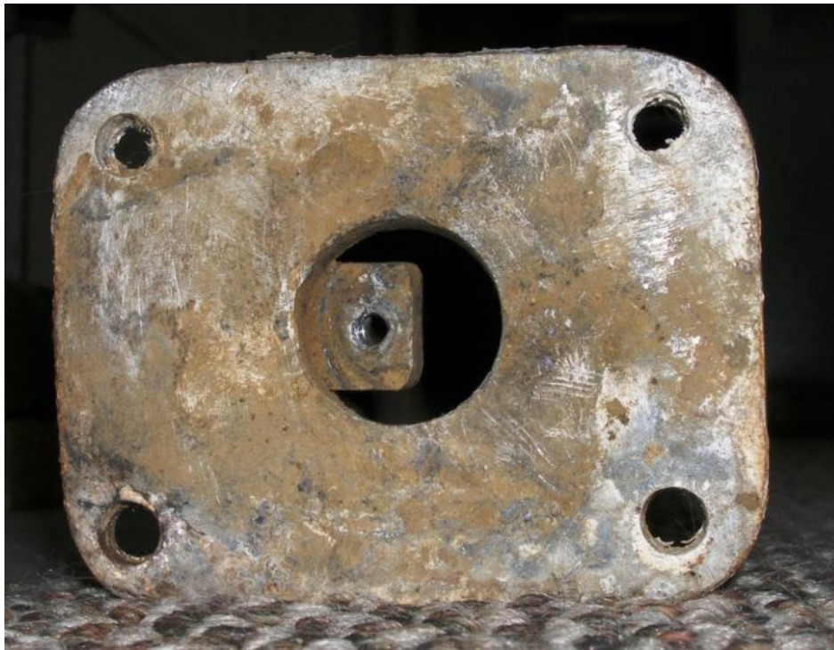
Foot of aluminum compression post. Note bonding tab for lightning ground wire to keel bolt.
