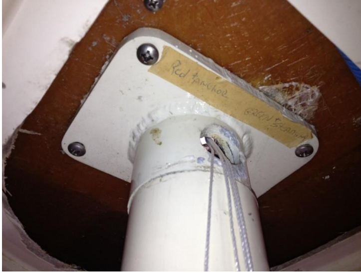
Upper post flange with wiring and mast removed. Post was removed and painted with two-part paint. Perfection I think it was. Color match was perfect.
