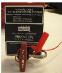
Figure #5: Pull Handle with Safety Pin and Tie
